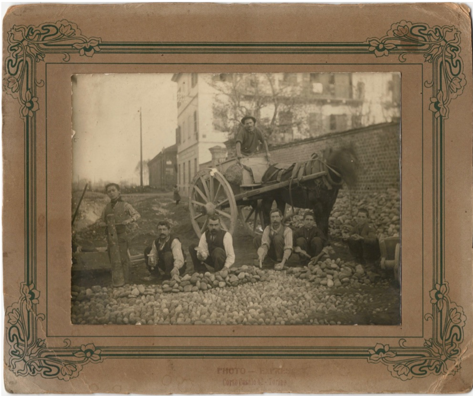
[Streeters] 1900s Turin Italy Construction Workers Make Cobblestone Street Cabinet Card. $60
